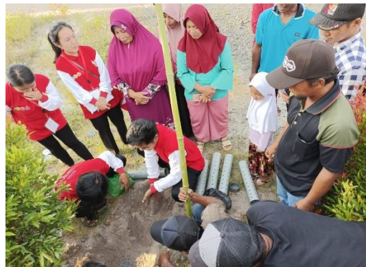
Gambar 9. Proses penimbunan pipa biopori
