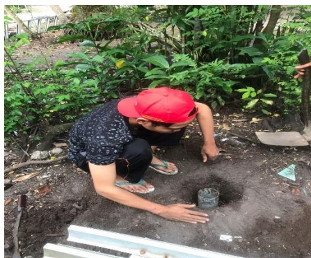
Gambar 7. Proses dipasangnya pipa biopori
