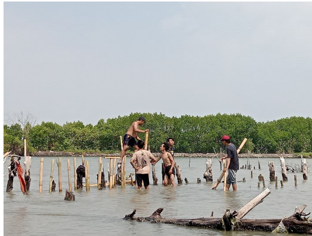
Gambar 5. Proses Finishing Bamboo Submerged Breakwater
