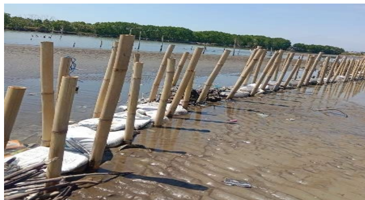
Gambar 6. Proses Pemeliharaan Bamboo Submerged Breakwater
