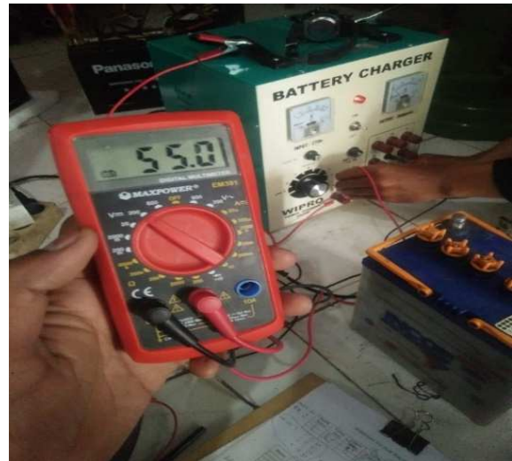
Gambar 6. Mengukur Voltase Charger Baterai
