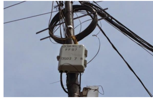
Gbr. 2 Perangkat ODP outdoor (Optical Distribution Point)
