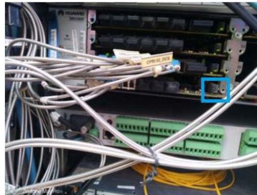
Gambar. 17 Pengecekan lampu idikator board WBBP
