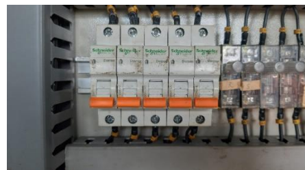
Gambar 10 MCB RST, Sirine, Voltmeter
